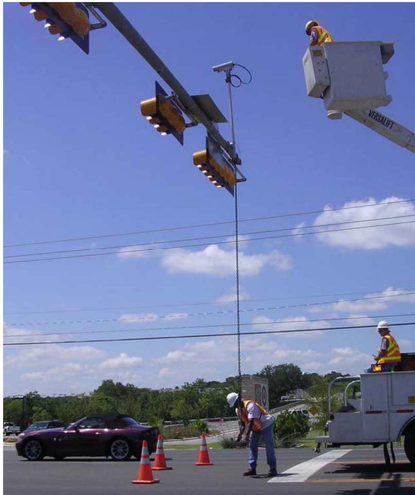
Figure 4.1: Static Load Test
