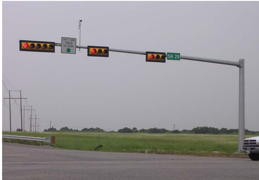
Figure 1.3: Typical Cantilevered Traffic Signal Structure in Texas
