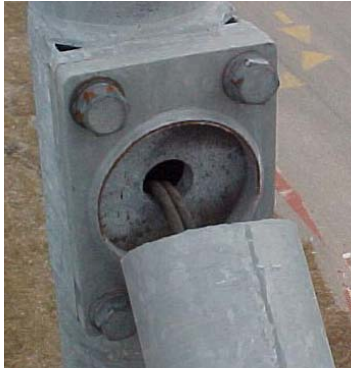
Figure 1.2: Fatigue Crack Initiated by Cyclic Loading
